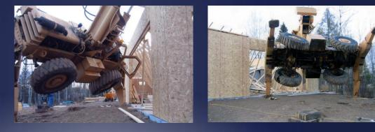
Pictures from crane accident – crane fell on Enercept SIP wall. Trusses collapsed but Enercept wall remained in tack.
