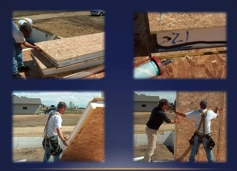
STANDARD WALL PANEL BEING INSTALLED
